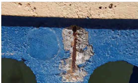
Figure 2-5: Spalling
