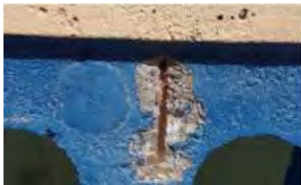
Figure 5 – Spalling
