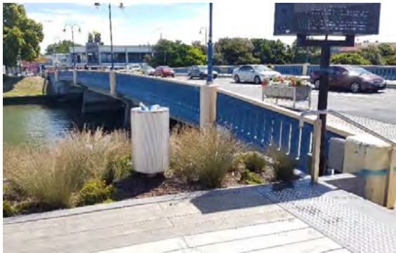
Figure 2-3: View from north
