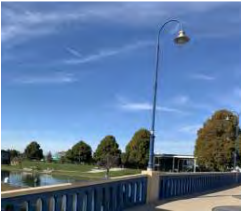
Figure 7 – Existing lamp posts
