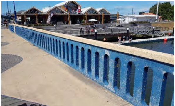
Figure 2-4: View from bridge
