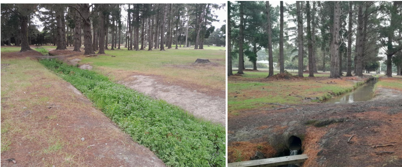
Figure 5. Water race in 2024 with an overgrowth of waterweed and a crossing in the distance (left) and another crossing adjacent to an informal, plank crossing further east.
