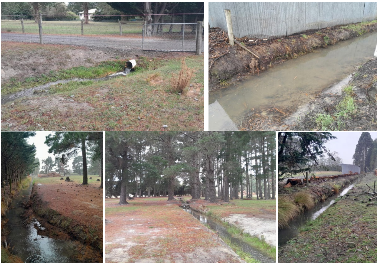
Figure 6. The water race enters the site through a culvert (top left) and has a silt substrate (top right) and generally bare banks, particularly where the race is shaded by pine trees or the shelter belt at the eastern boundary.
