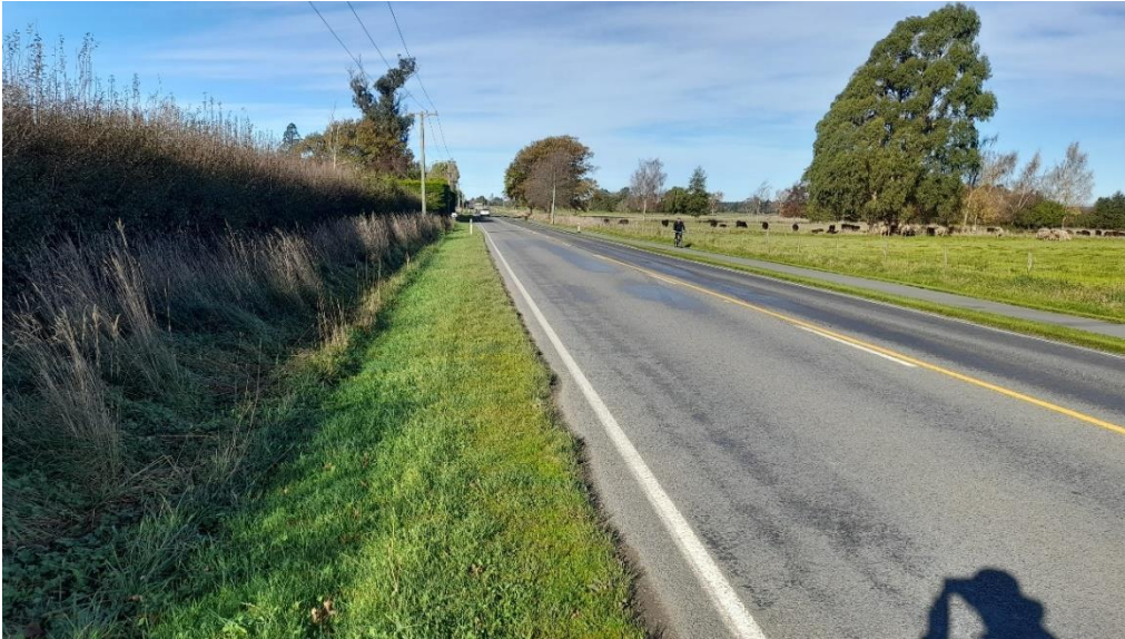
Photograph 3-1: Rangiora Woodend Road, Looking East Along Site Frontage
