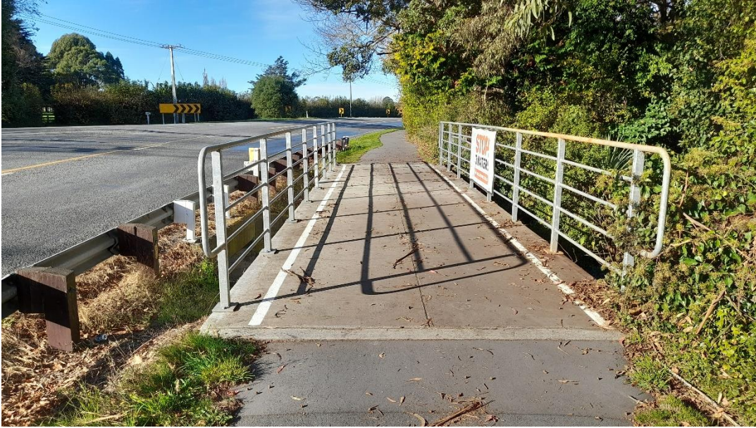
Photograph 3-14: Rangiora Woodend Path Bridge at Cam River
