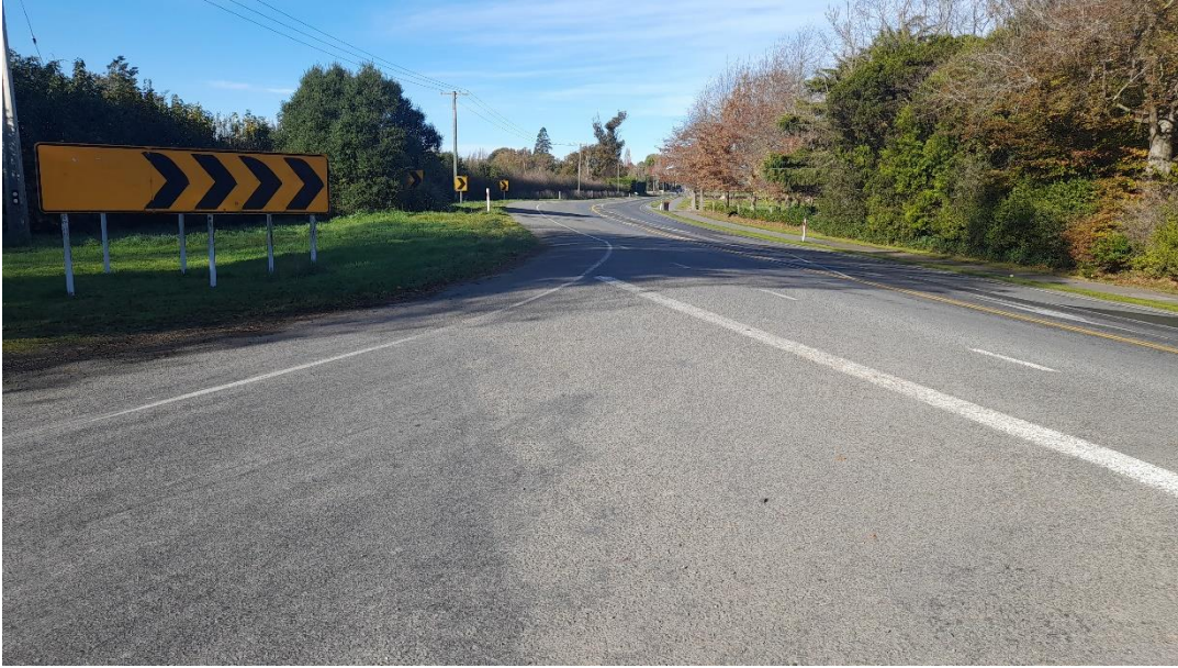
Photograph 3-7: Sightline to Left at Rangiora Woodend Road / Golf Links Road Intersection
