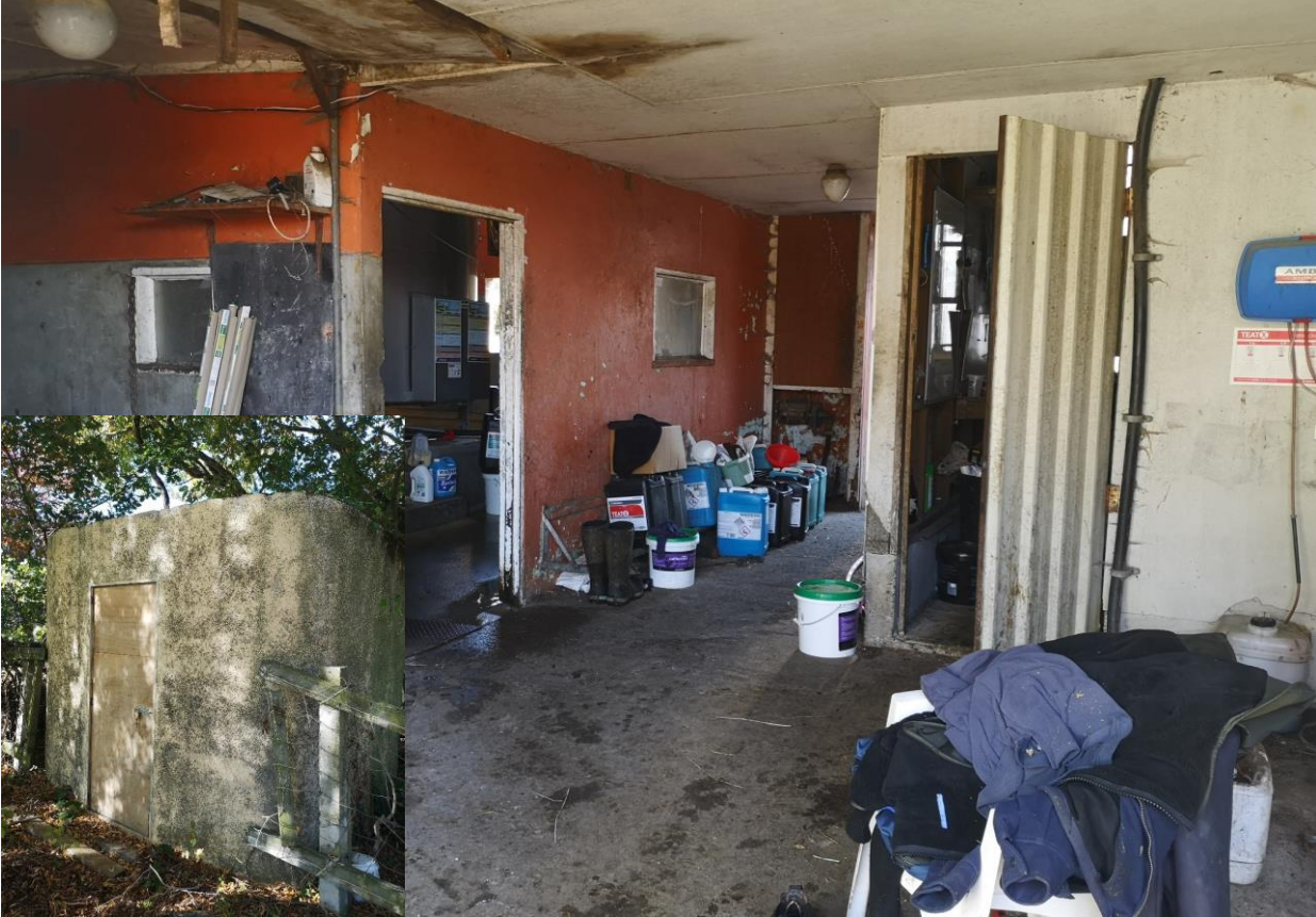
Photograph 5: Chemical storage area. Inset: Storage shed within the site.
