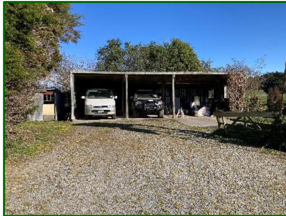
Photo 3 – Timber & pole shed with concrete floor
