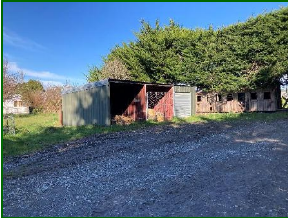
Photo 8 – Iron & timber shed
