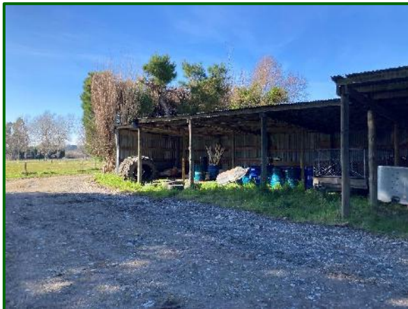
Photo 4 – Iron & timber shed with oil drums
