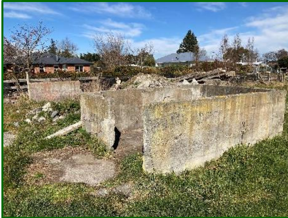
Photo 24 – Remains of concrete building
