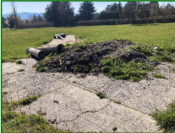
Photo 26 – Concrete pad with gravelly soil, concrete pipes
