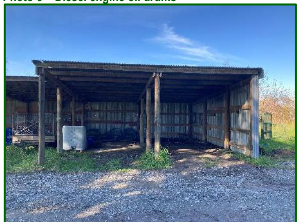
Photo 7 – Iron & timber shed
