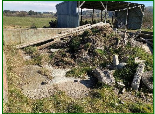
Photo 25 – Soils, timber and concrete within building remains
