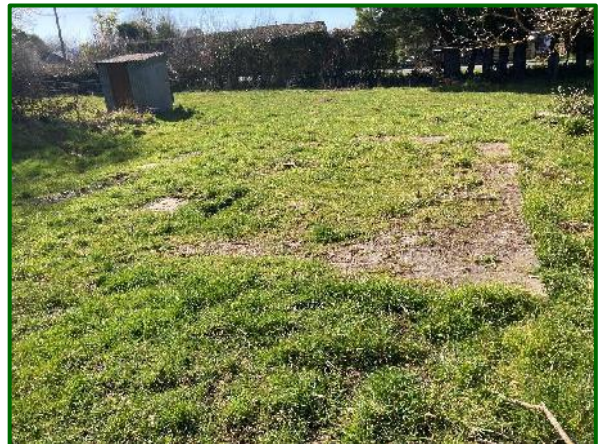
Photo 29 – Concrete pad and pump shed
