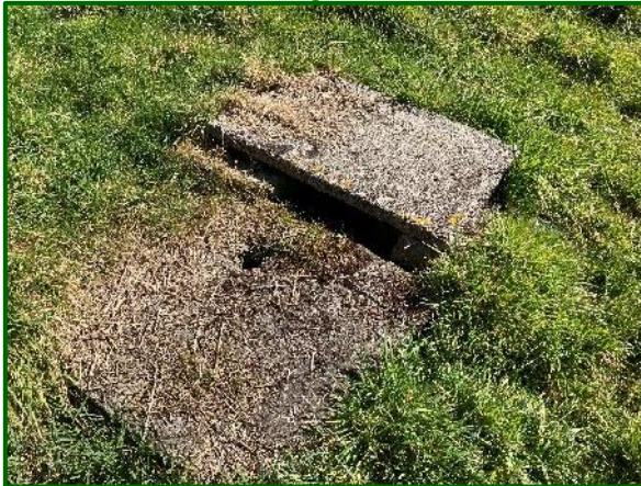
Photo 32 – Concrete well cap
