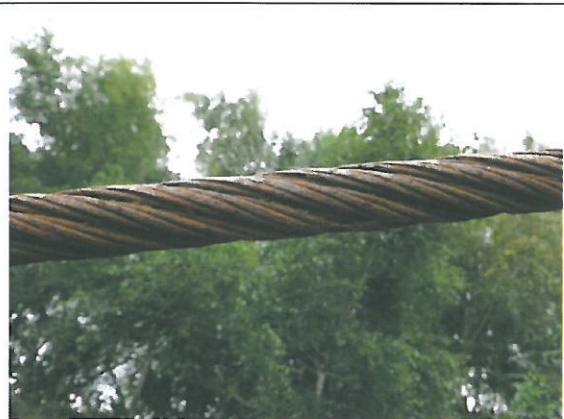
Photograph 6 – Wire Rope Connection
