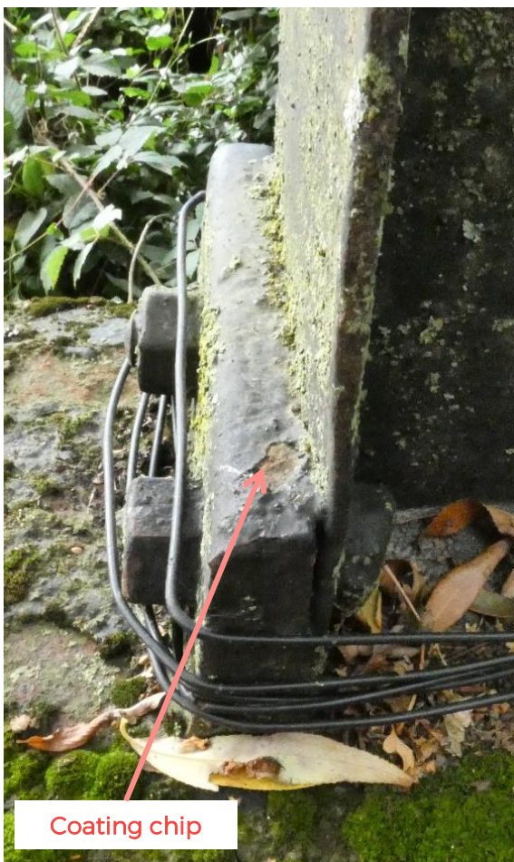
Figure 6.3: Chip in unidentified black coating on west tower
