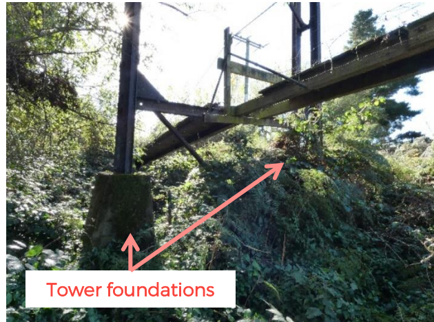
Figure 5.6: Tower foundations - eastern tower
