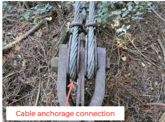
Figure 4.5.2: Eastern upstream cable anchorage connection
