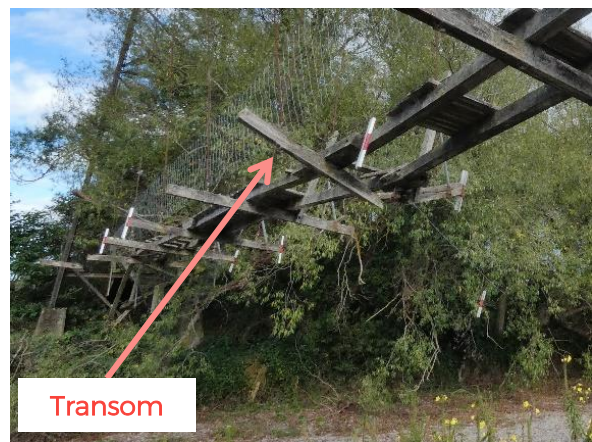
Figure 4.1.6: Transom failure
