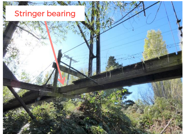
Figure 1.2: East abutment stringer bearing
