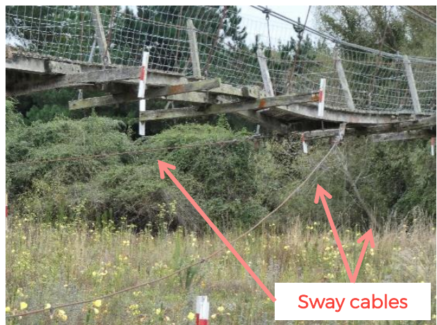
Figure 3.14: West abutment sway cables
