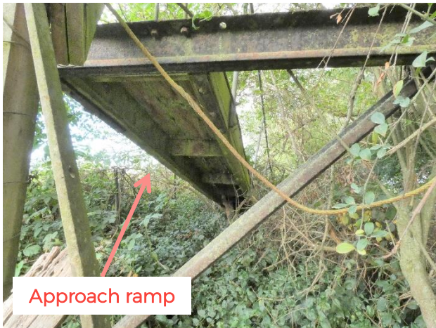
Figure 1.10: West approach ramp - underside
