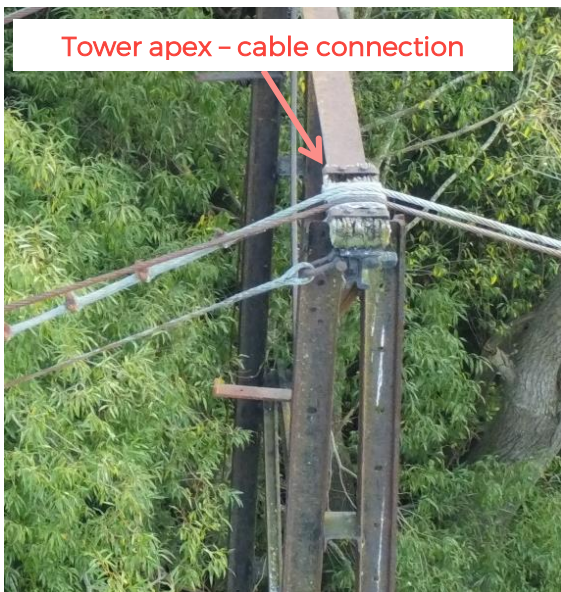
Figure 3.7: Cable tower connection - west abutment - downstream side
