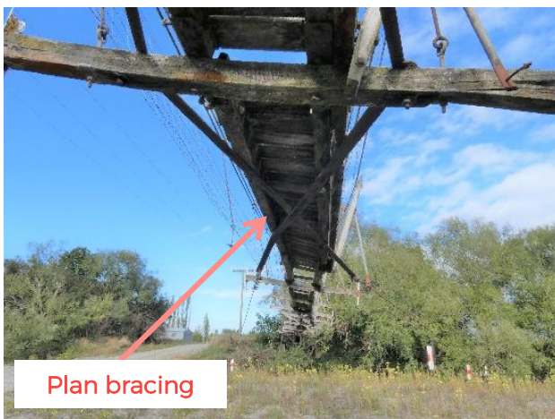
Figure 4.4.1: Plan bracing facing the western abutment
