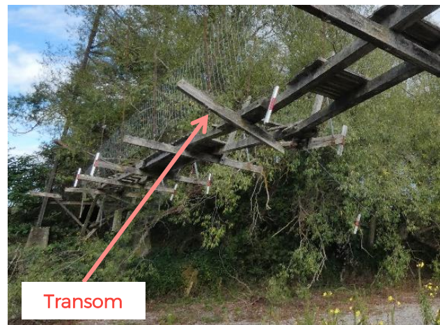
Figure 1.7: Transom failure
