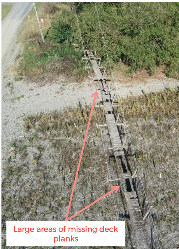
Figure 4.1.1: Deck plank condition overview – facing west abutment
