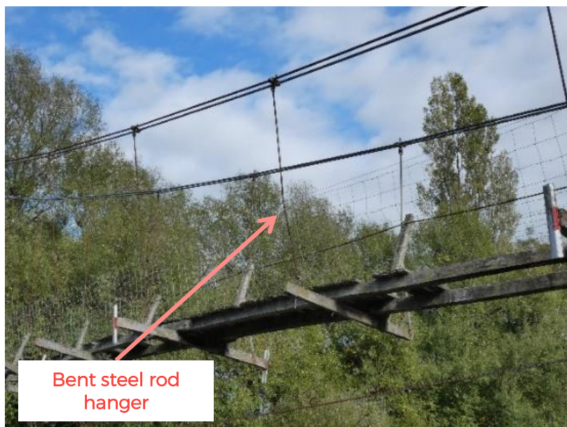
Figure 4.2.3: Bent steel rod hanger
