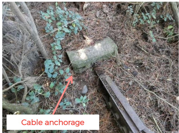
Figure 4.4: Eastern upstream cable anchorage block
