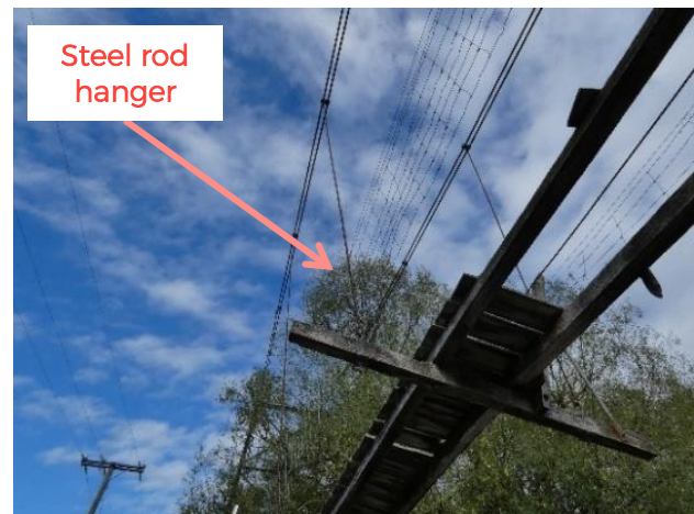
Figure 2.2: Typical steel rod hanger
