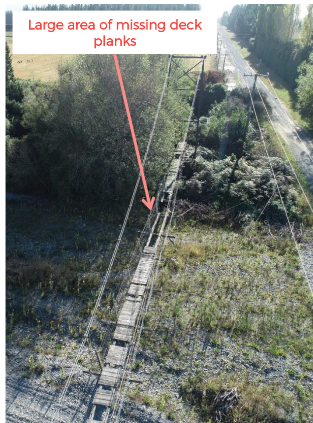
Figure 4.1.2: Deck plank condition overview – facing east abutment
