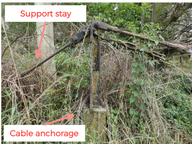
Figure 4.5.3: Western downstream sway cable anchorage
