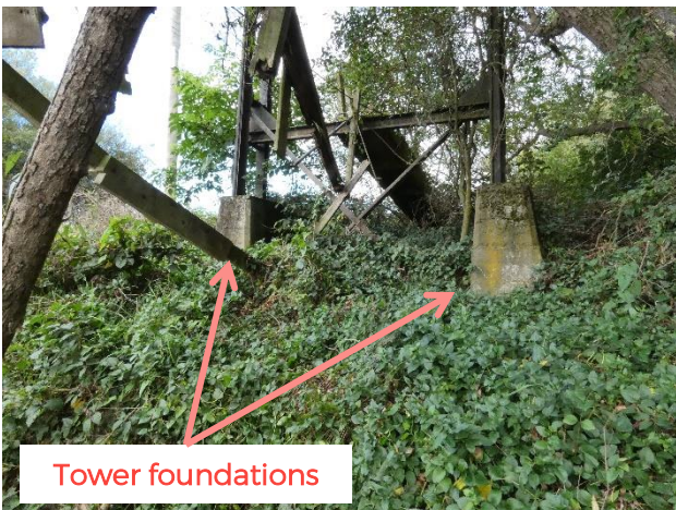
Figure 4.6.2: Tower foundations – western tower
