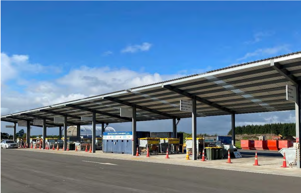
Figure 3-3: Pines RRP covered podium
