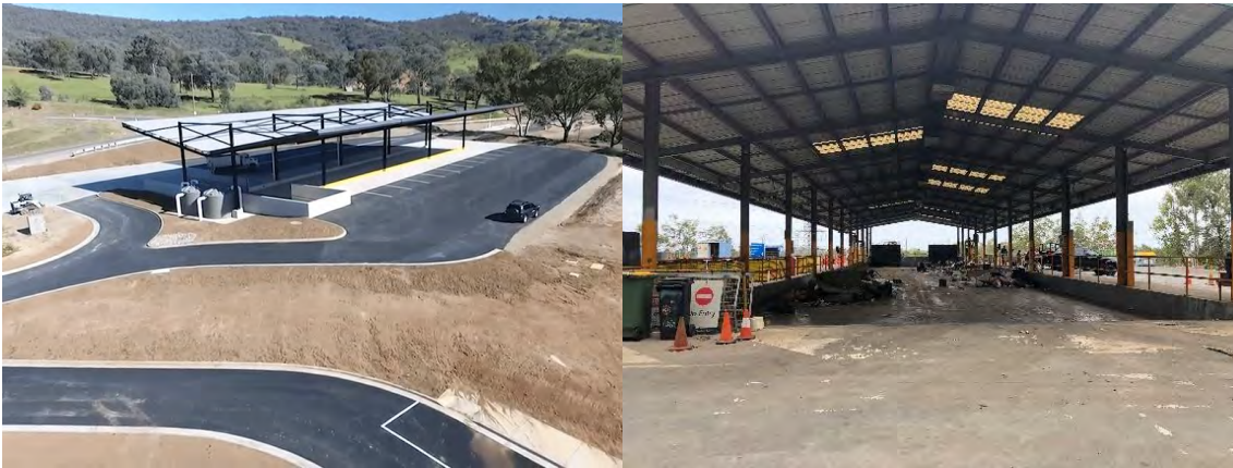
Figure 3-7: Facility Examples (Albury Residual Waste Facility, Molendinar shallow Residual Waste Push Pit).
