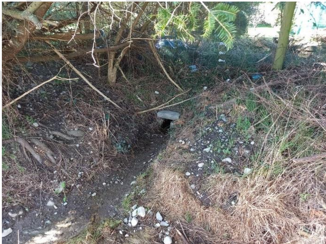
Figure 1: Swale Entrance into 55A Burnett Street
