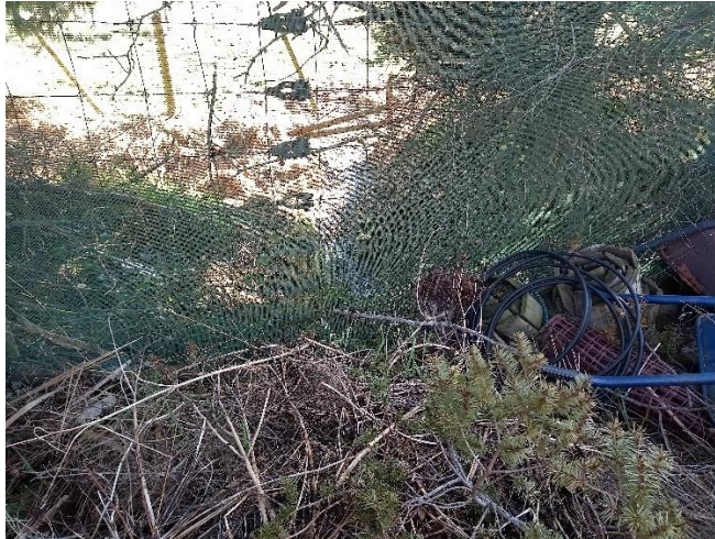
Figure 7: Looking at swale entrance from 55A Burnett Street into A&P Showgrounds
