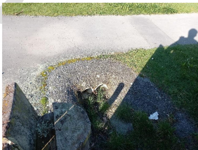
Figure 9: Piped Swale Outlet 53 Burnett Street
