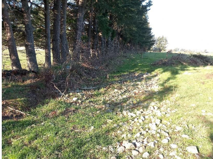
Figure 10: Swale at rear of 160 High Street
