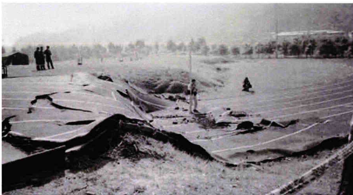
Figure 9 Fault scarp formed on the Chelungpu Fault during the magnitude 7.6 Chi-Chi Earthquake, Taiwan, 1999. The disrupted running track shows damage typical of a reverse fault ground-surface rupture. This location lies on a stream terrace that is younger than the previous rupture event on the fault, so that there was no scarp here before the earthquake. This example illustrates the sorts of effects that can be expected on active reverse faults of the Waimakariri District the next time any particular fault experiences a surface rupture earthquake. Photo and information from Kelson et al. (2001).
