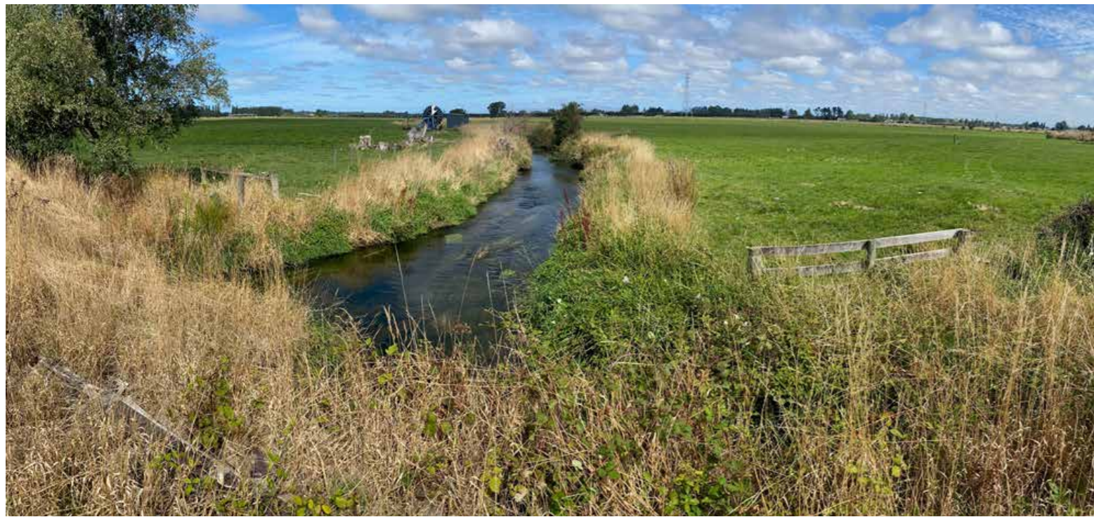
Site Photograph : Looking south over North Brook from Boys Road
