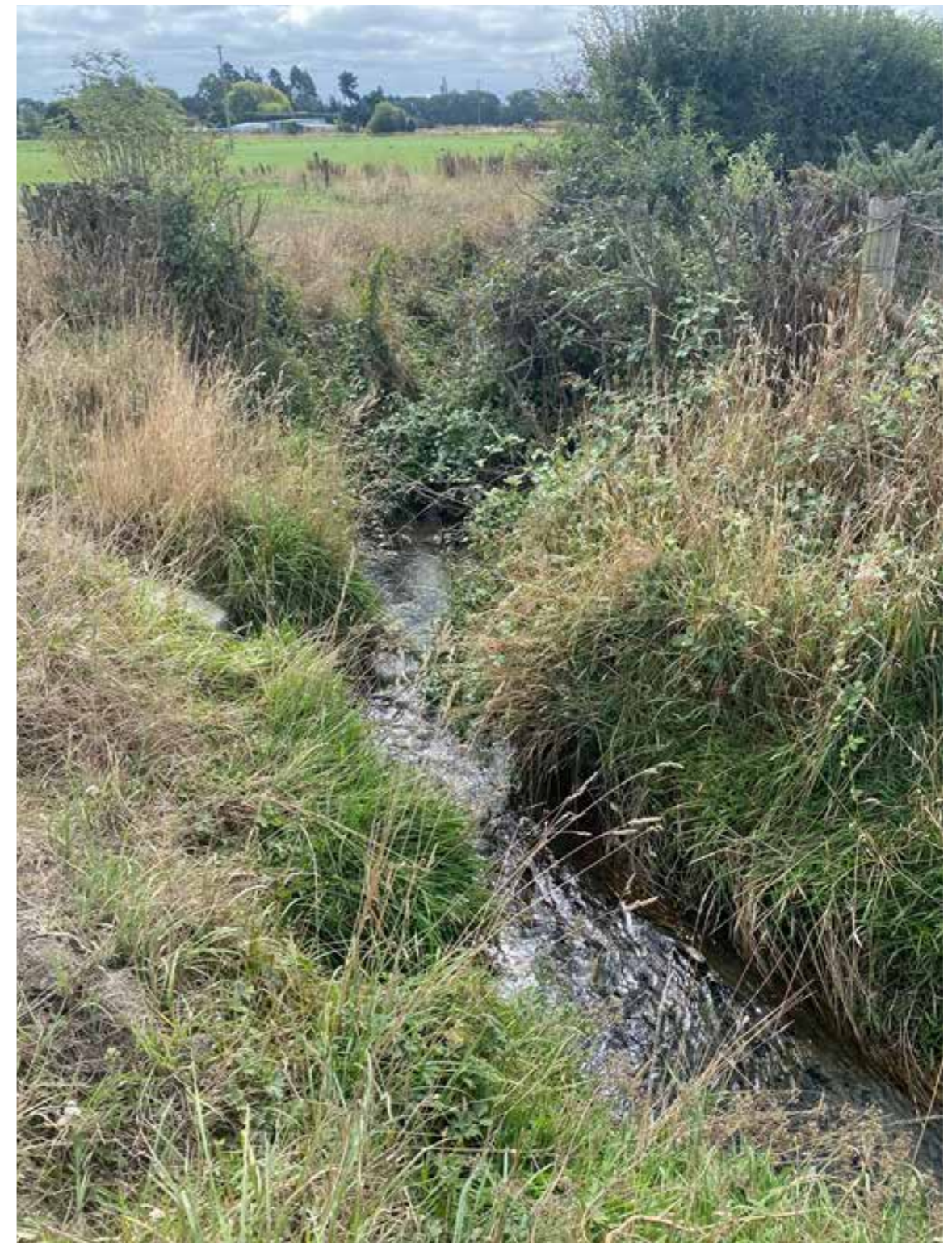
Site Photograph : The Middle Brook at Marsh Road
