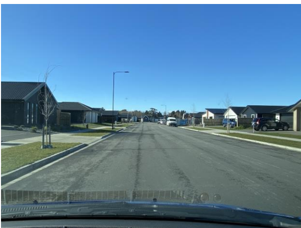
Figure 5 - Completed Houses within Woodland Estate
