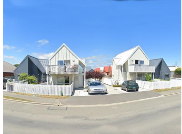
Figure 2- Rangiora Housing New Zealand Multi Lot Development (High Street)
