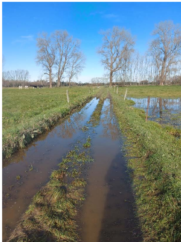
Figure 5: Surface water ponding within the farm track.
