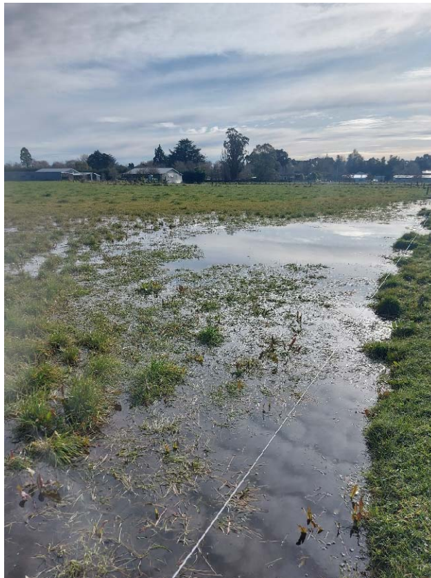
Figure 4: Surface water ponding associated with farm track.
