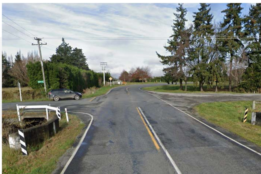
Photograph 4: Cones Road / Dixons Road Intersection Looking South
