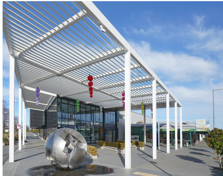
Kaiapoi Service Centre
