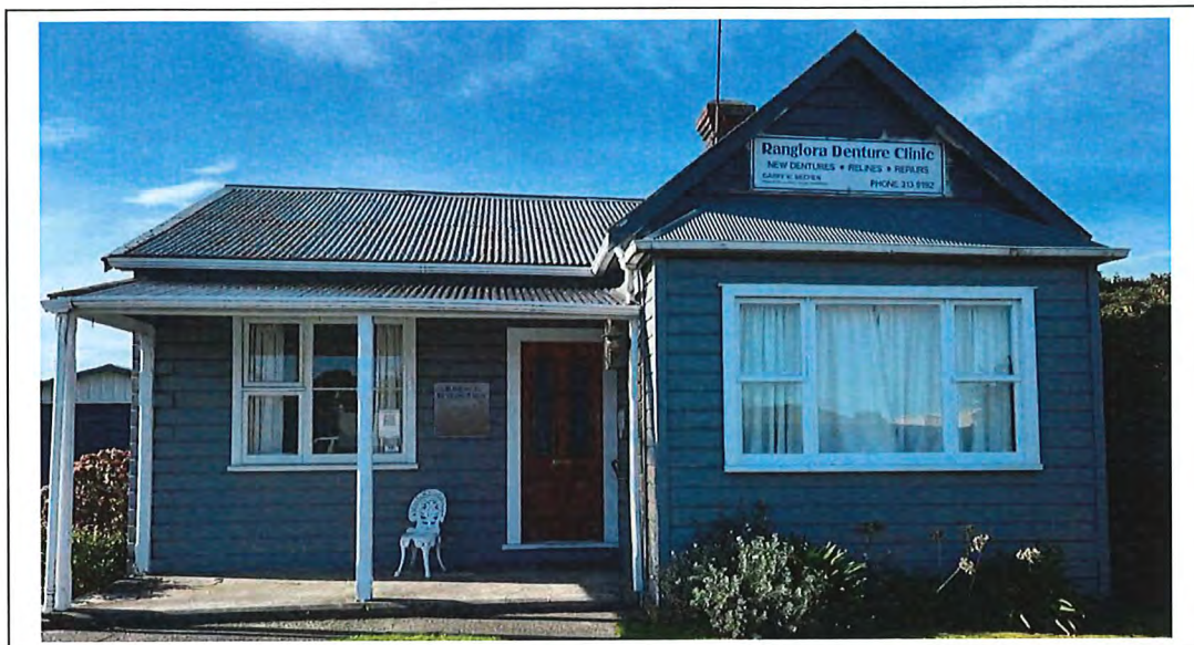
House, 38A Ashley Street, Arlene Baird, 13 May 2022, Heritage New Zealand Pouhere Taonga
