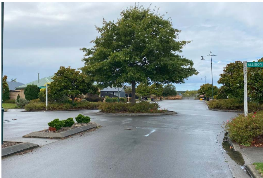
Photograph 8: Magnolia Boulevard / Allison Crescent / Fergus Street Roundabout Looking East
