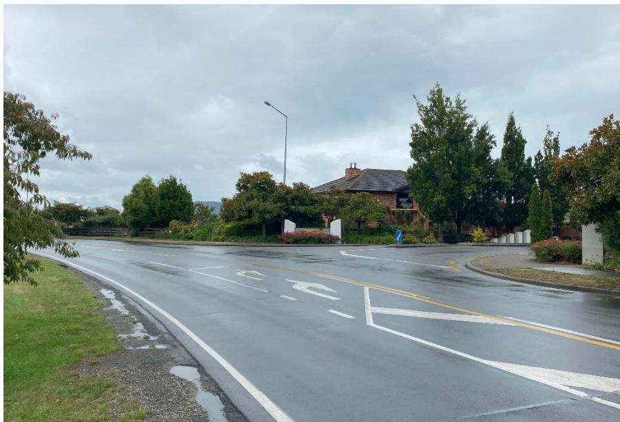
Photograph 10: Williams Street / Magnolia Boulevard Intersection Looking North
