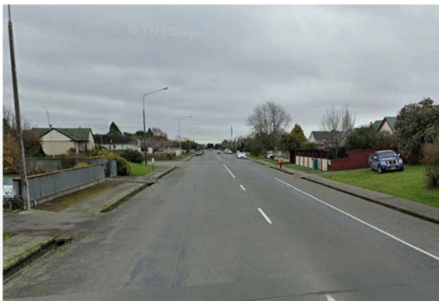
Photograph 11: Typical Cross-Section of Williams Street Looking North
