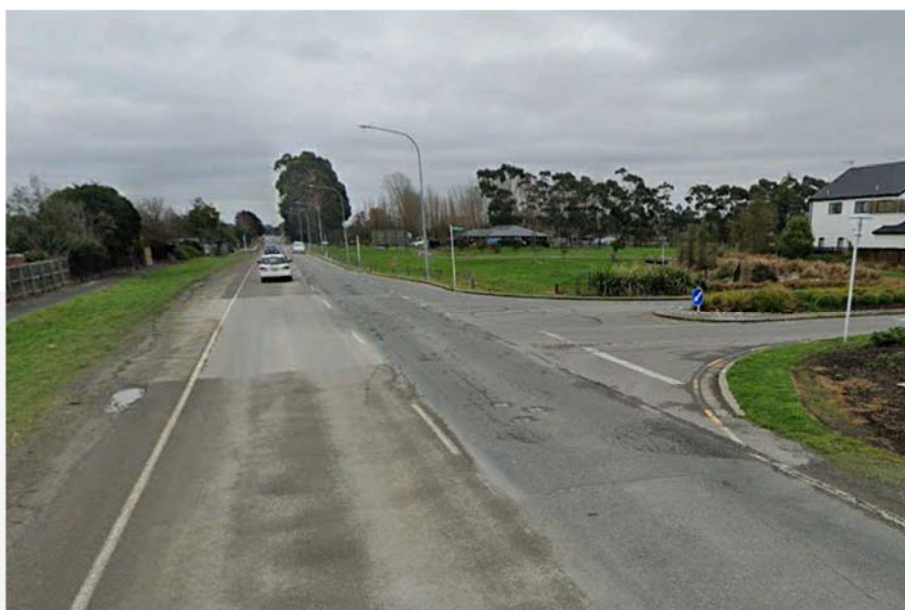
Photograph 15: Beach Road / Tuhoe Avenue Intersection Looking West
