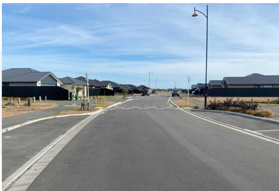
Photograph 13: Isa Lei Road Looking North
