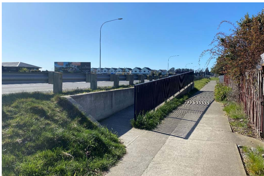
Photograph 19: Ramp Connection to Beach Road Shared Route
