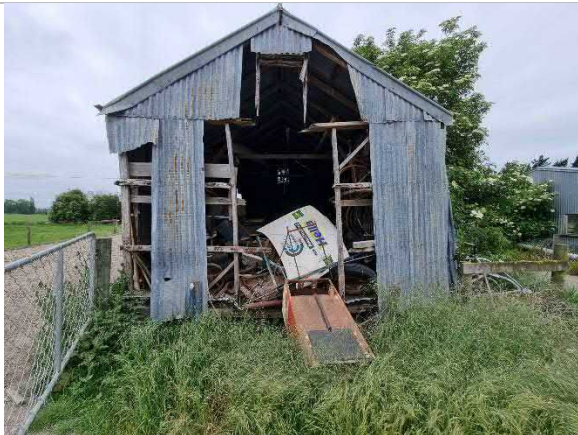
Photo 15: Scrap metal storage along the eastern side of the site.
