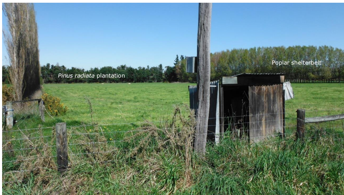
Photo 3. Power pole and disused well shed at 81 Gressons Road (looking south).
