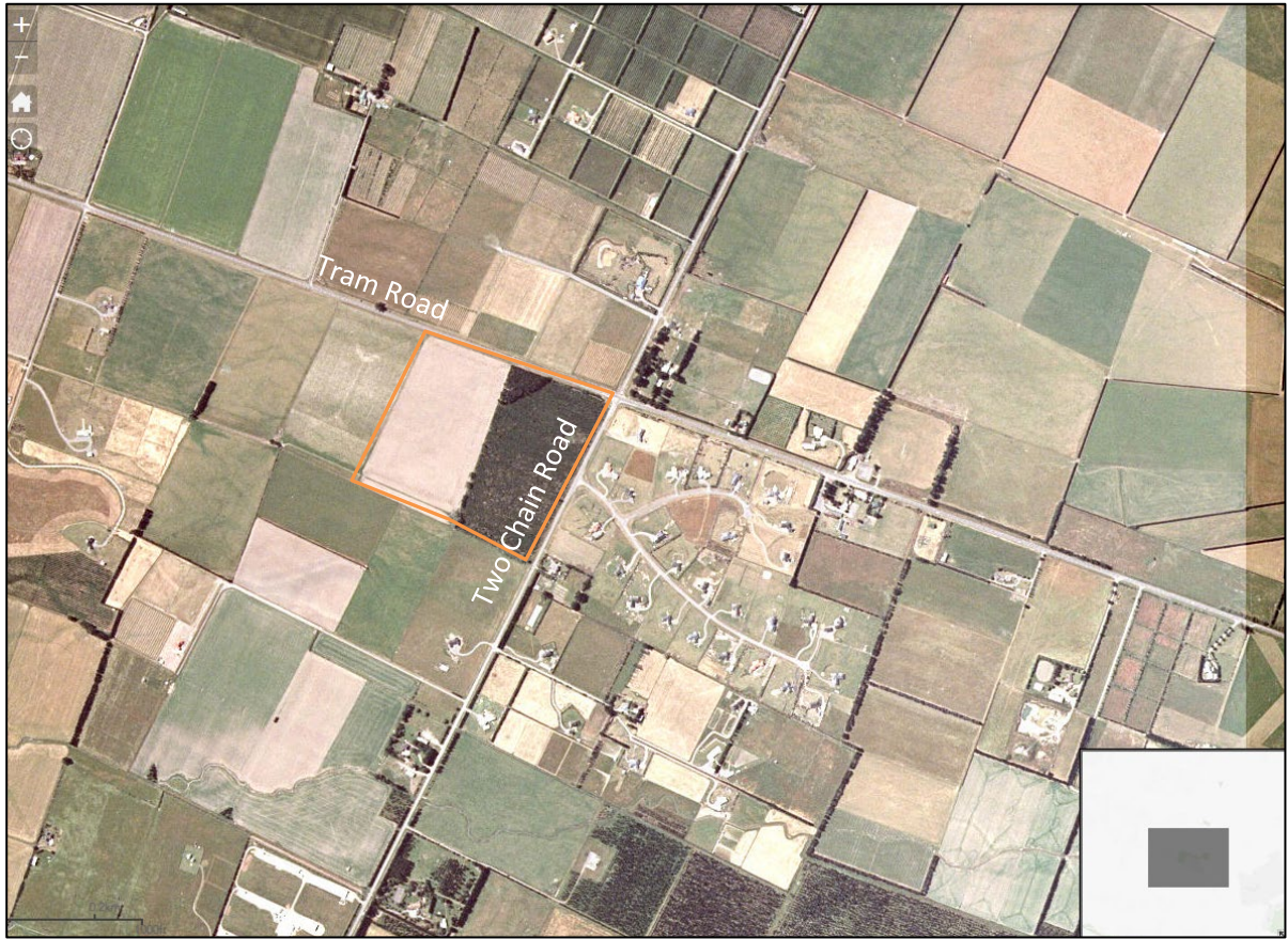
Photograph 9: 2000-2004: Block A - 1401, 1419 and 1379 Tram Road, Swannanoa indicated by orange outline (Source Canterbury Maps).
