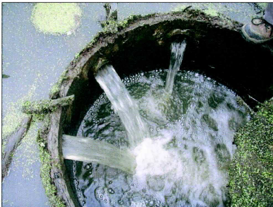
Plate 2-7 Taerutu Gully to old Taranaki Stream Discharge - flow through PVC Pipes (~10l/s)
