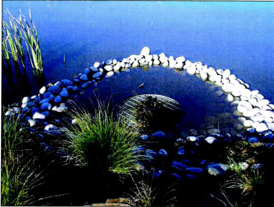
Plate 2-1 Orifice weir which discharges from Taerutu Gully to old Taranaki Stream
