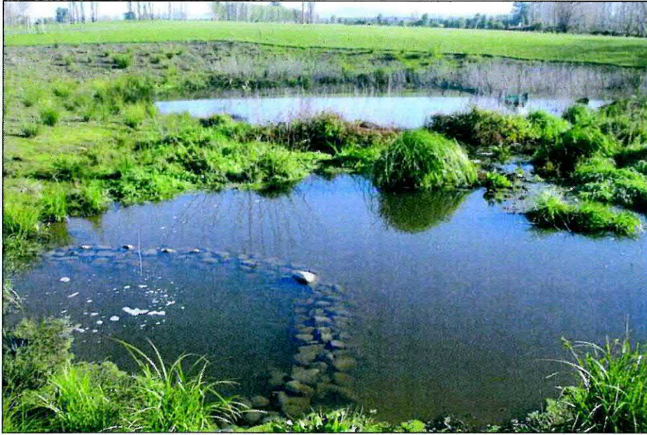
Plate 2-2 Taerutu Gully to old Taranaki Stream discharge, rock filter, and fabric filter
