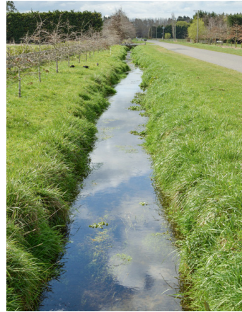
An example of a well maintained drain with good vegetation cover on the banks.
