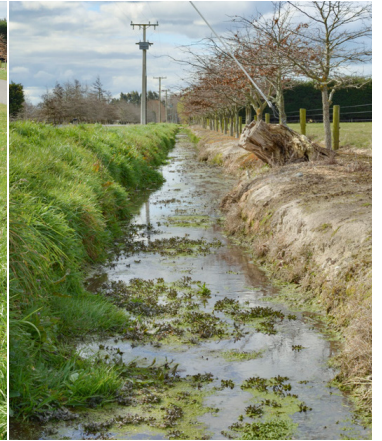
An example of a poorly maintained drain with over-sprayed vegetation which is causing bank instability.
