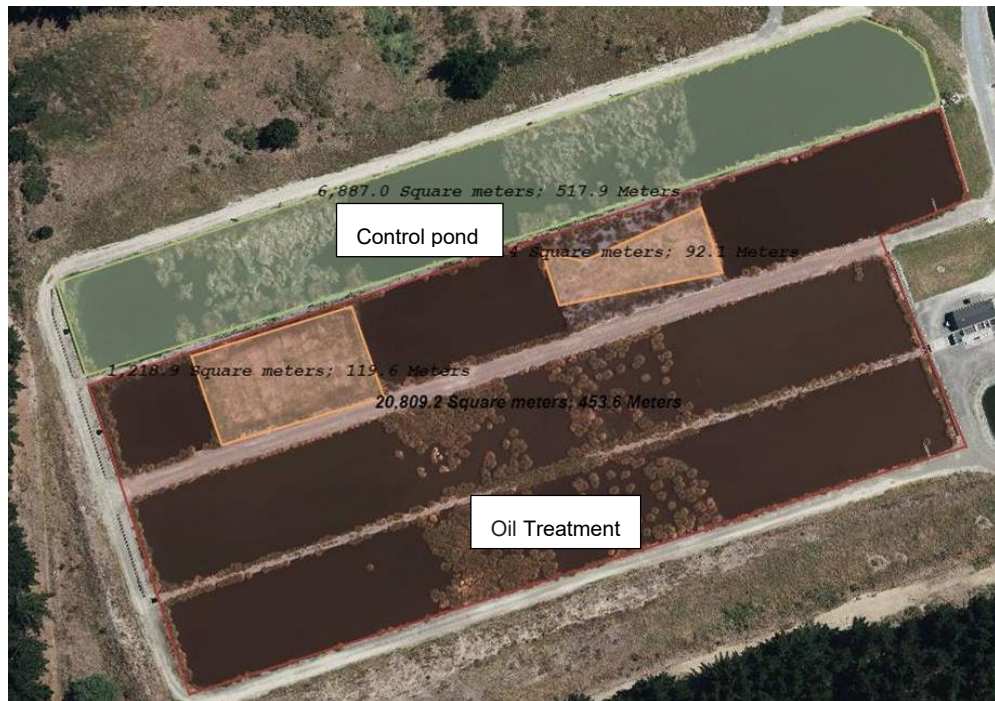
Figure 4: Control and treatment areas for the vegetable oil trial at Woodend WWTP. The orange areas are not sprayed as there are dense plantings with little open water midge habitat.
