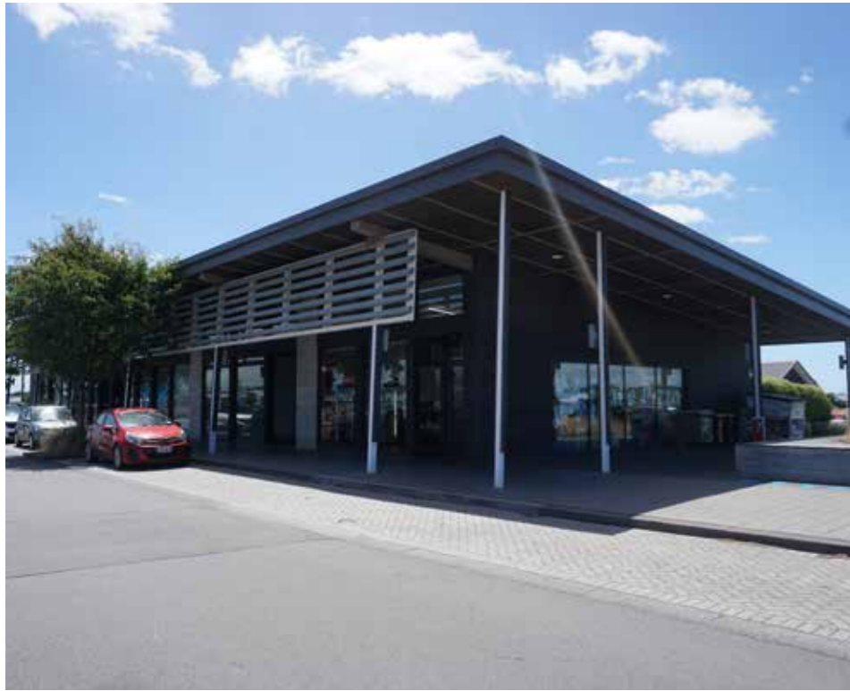
A Pegasus commercial strip within Pegasus' urbanised centre overlooking public open space on Pegasus Main Road with parking in front
