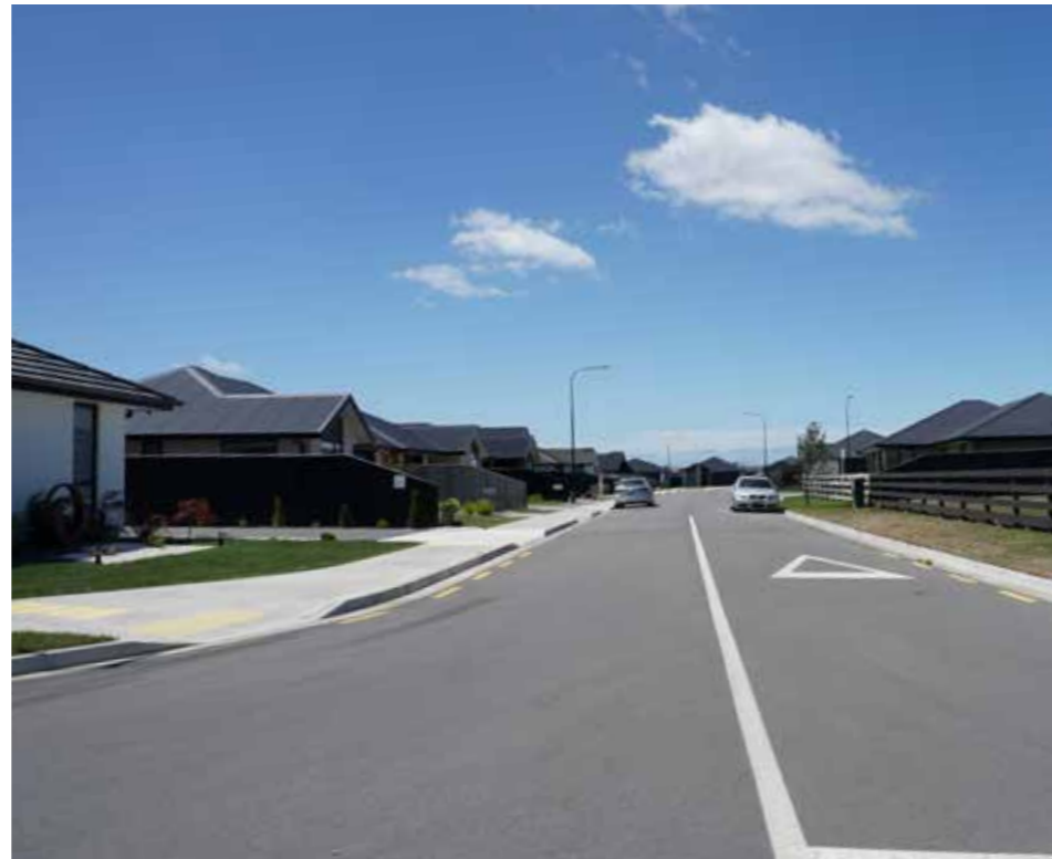
E Woodend residential dwellings are predominantly single-storey with an increasing number of modern development with open or semi-open frontage and good street connection.
