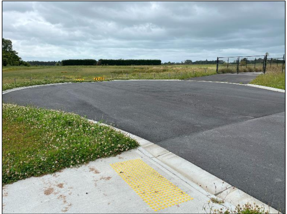
Photograph 5-10: Lorrimer Street turning head
