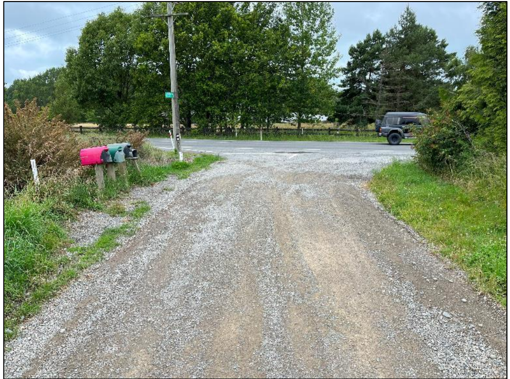
Photograph 5-7: Wards Road approach to SH1
