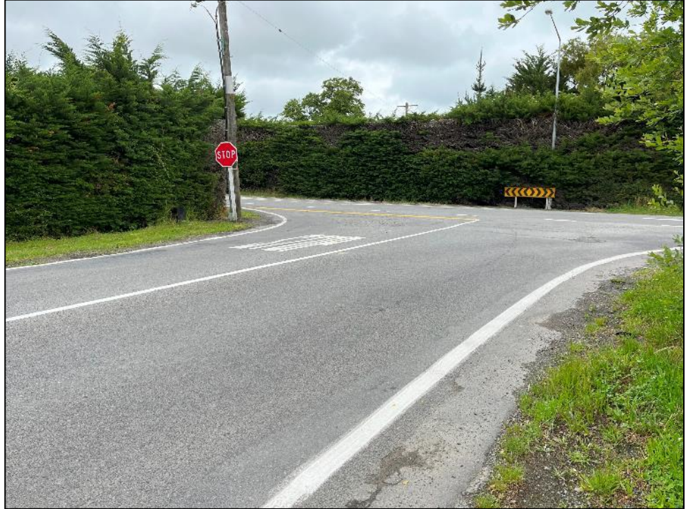
Photograph 5-3: Gressons Road approach to SH1
