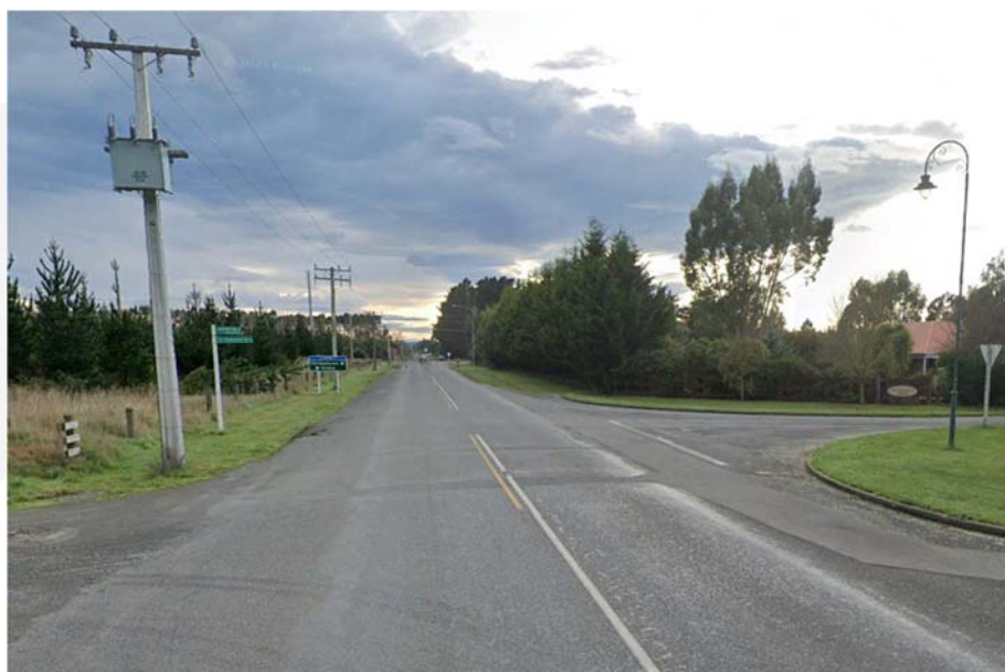
Photograph 4: Two Chain Road/ Winter Road Looking North (Western Site on Left)
