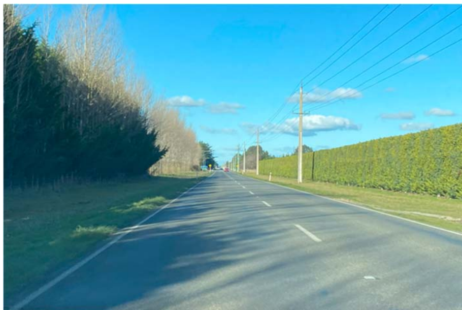
Photograph 1: Tram Road West of Western Site, Looking East (Western Site on Right)
