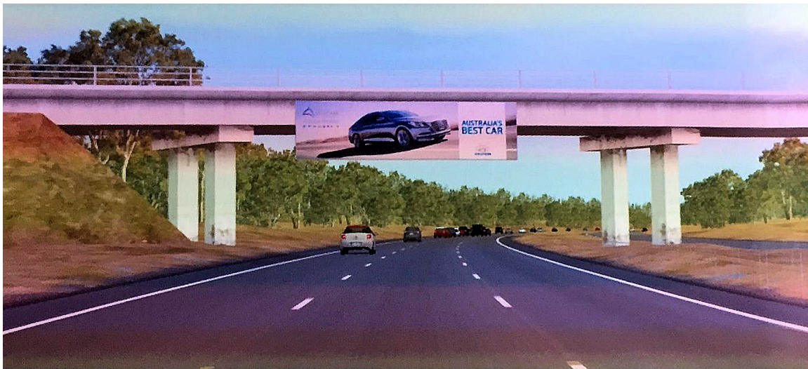
Fig. 3. Example of an overhead billboard on a bridge.
