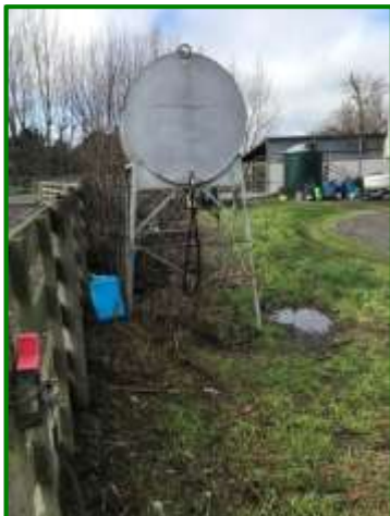
Photo 16 – Above ground diesel tank
