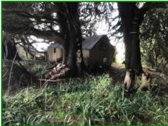
Photo 13 – Derelict chicken shed
