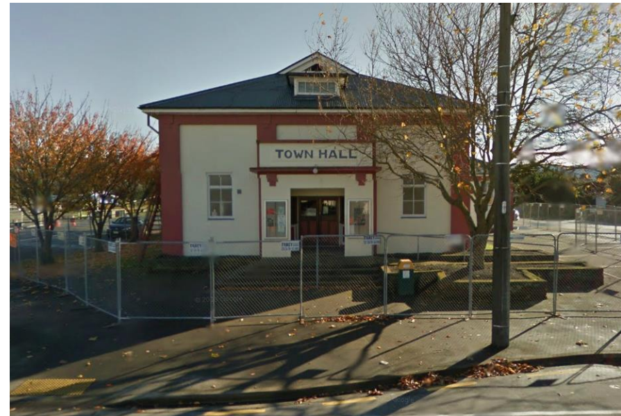
Figure 17. Oxford Town Hall prior to works, view from Main Street
