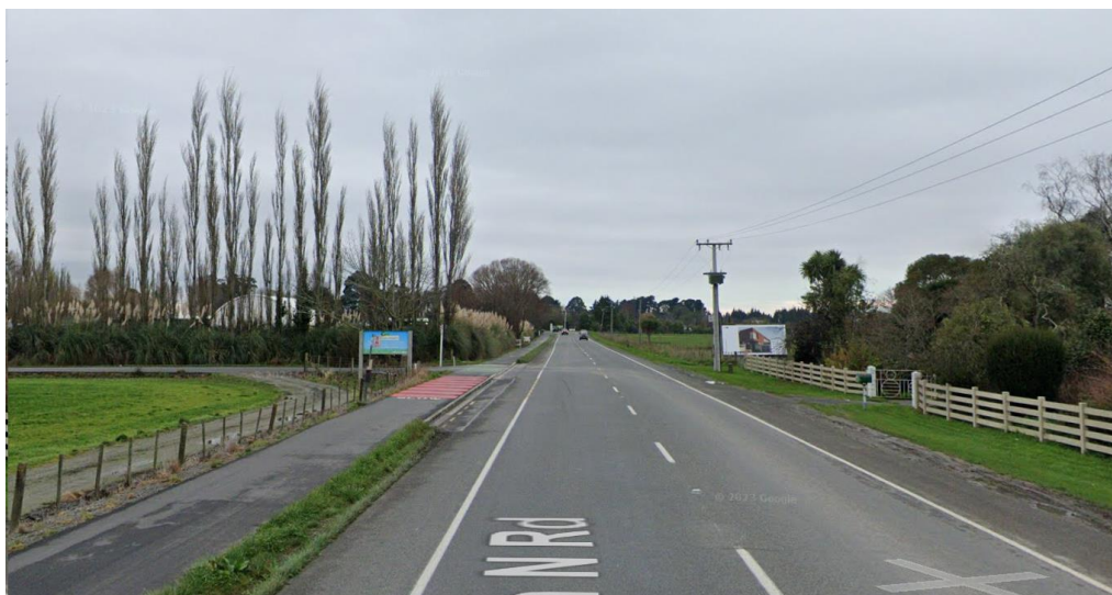
Figure 3: Main North Road looking north 2 .
