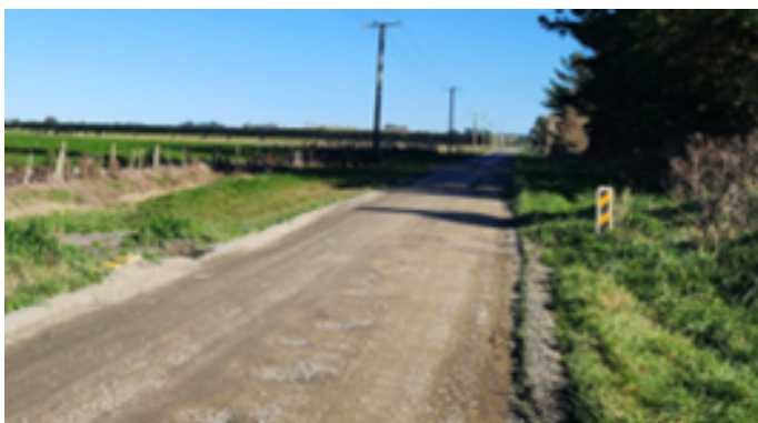
Figure 2. Ashworths Road looking west
