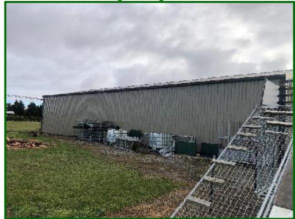
Photo 6 – Minor storage at rear of shed
