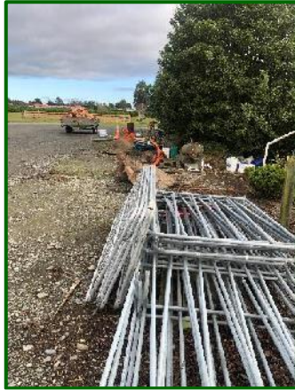
Photo 3 – Storage of fencing & digger buckets
