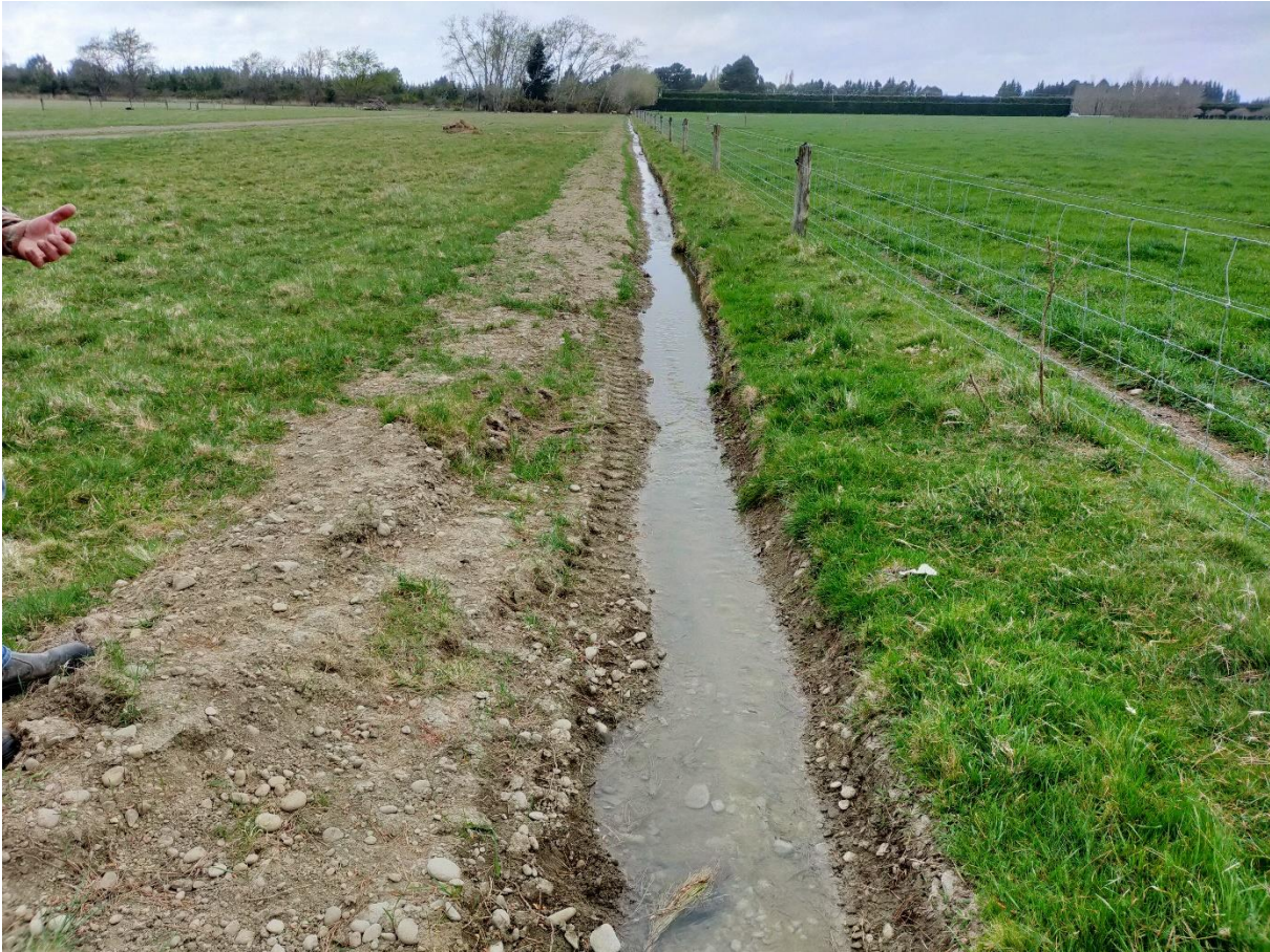
Figure 2 Recently realigned water race at southern edge of property boundary (photo taken during site visit on 22 nd September 2023)
