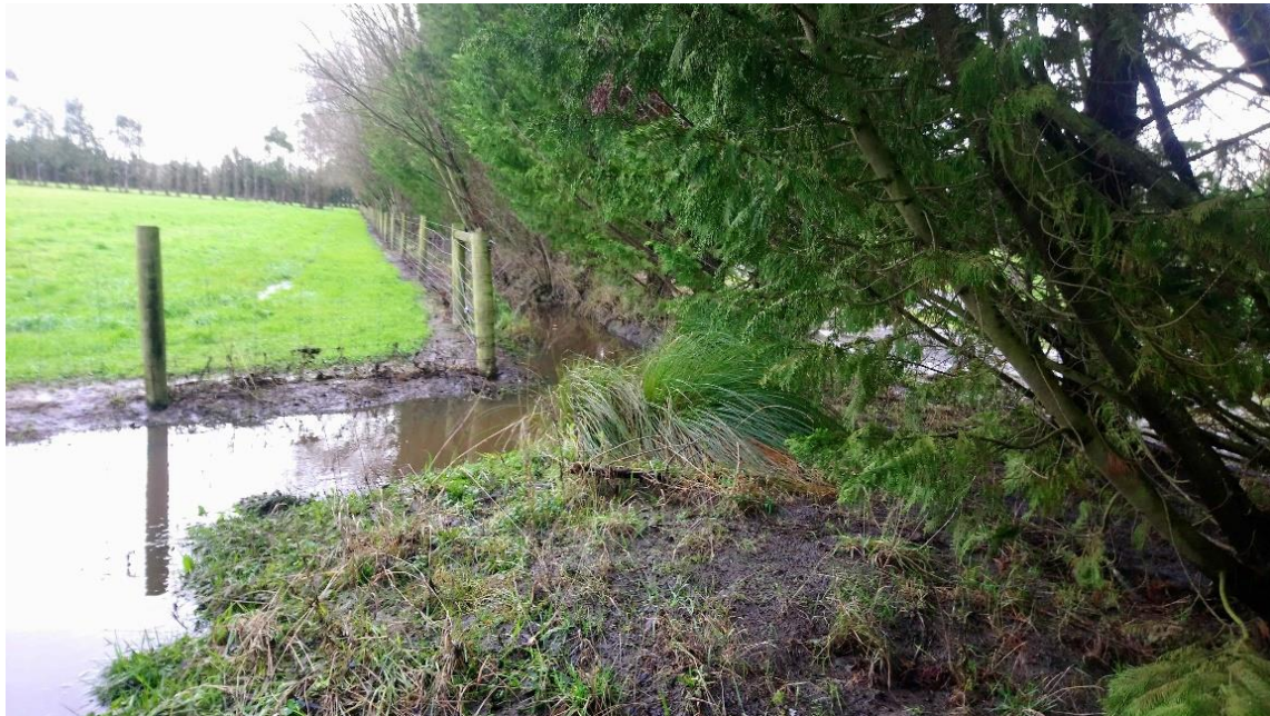
2. Jacksons Road – Example of Vegetation restricting drain flow and access for maintenance.
