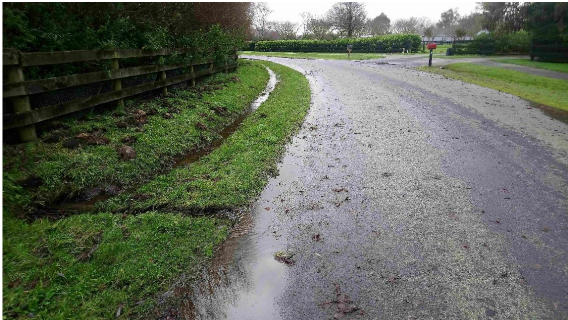
1. Wilson Drive - Build-up of turf in roadside swale preventing drainage of the carriageway
