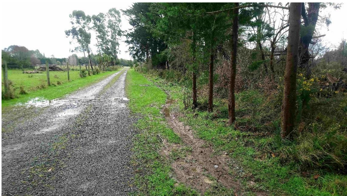
3. Jacksons Road – Example of poorly maintained section of drain, evidence of localised flooding of driveway.
