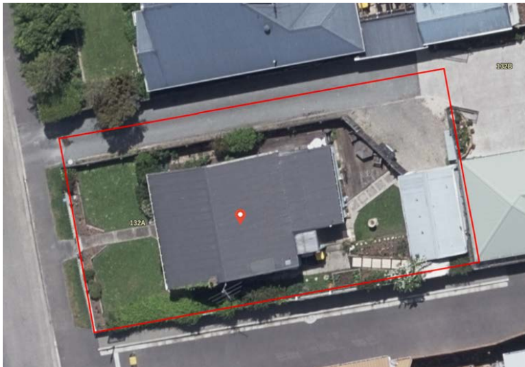
Extent of scheduling, former Rangiora Post & Telegraph Office, 132A King Street, Rangiora.
