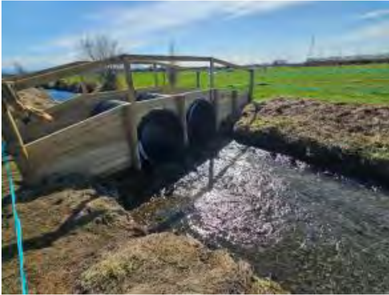
Figure 12 – A bridge made of 2 large culverts under construction. A large pool has formed just downstream of the outlet. To avoid water undermining the culverts, large cobbles could be placed in the bed immediately downstream of the pipes. This would also create instream habitat variation.
