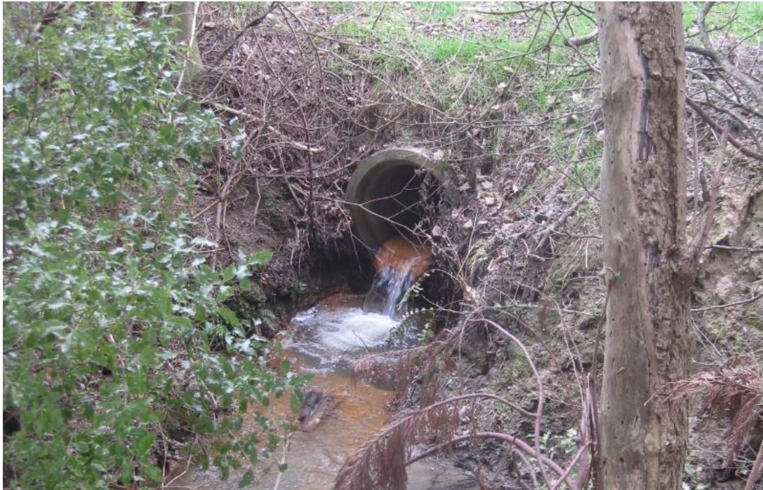
Photograph 2: The large drain situated on the neighbouring property, south of the site. (July 2012)
