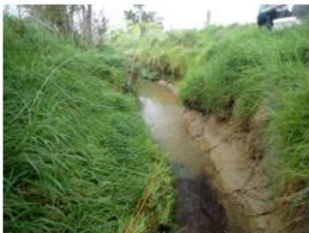
Figure vi. Looking downstream at Site 3 Frahams Creek. Deeply incised, firm clay substrate. Photo taken 26/09/2023.
