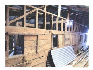
Significant deterioration to tongue and groove flooring throughout services/feed-store room makes accessing this area hazardous. Floor substructure appears largely sound and serviceable. Our proposal includes replacing this tongue and groove flooring.
