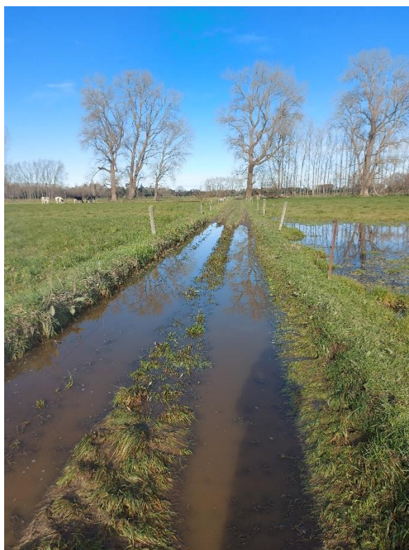
Figure 5: Surface water ponding within the farm track.
