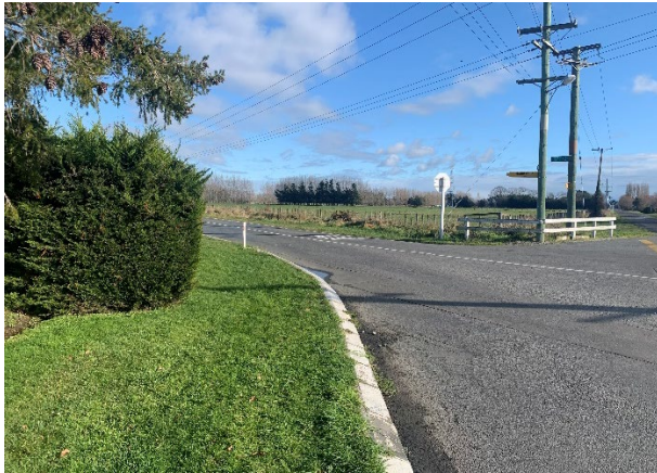
Figure 4: Left turn movement – long radius encouraging high turn speed
