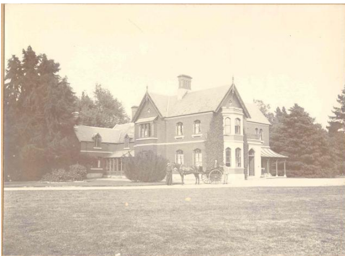
Homestead as built.
