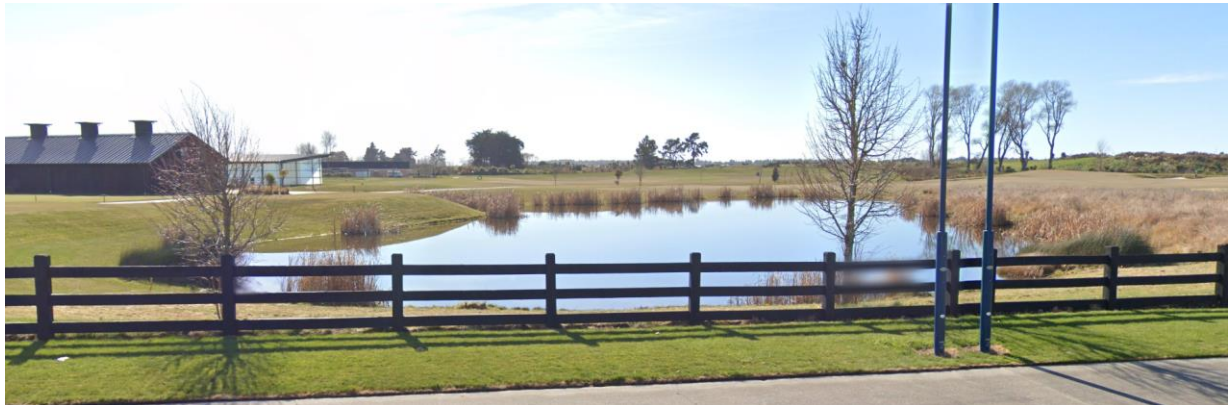
Figure 2: View of constructed amenity pond (image care of Google Streetview, captured August 2019)
