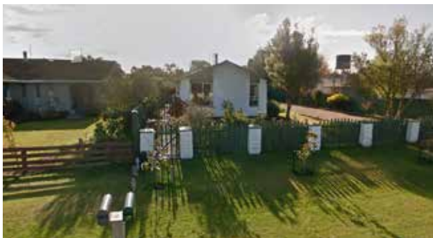
Residential 3 Zone example: houses on Canterbury St, Ashley.
