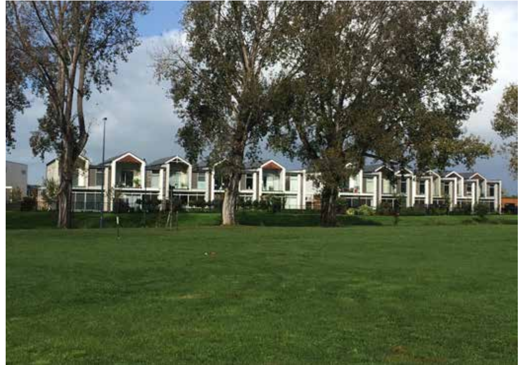
Residential 7 Zone example: new terraced houses overlooking the Kaiapoi River, Silverstream., Silverstream.
