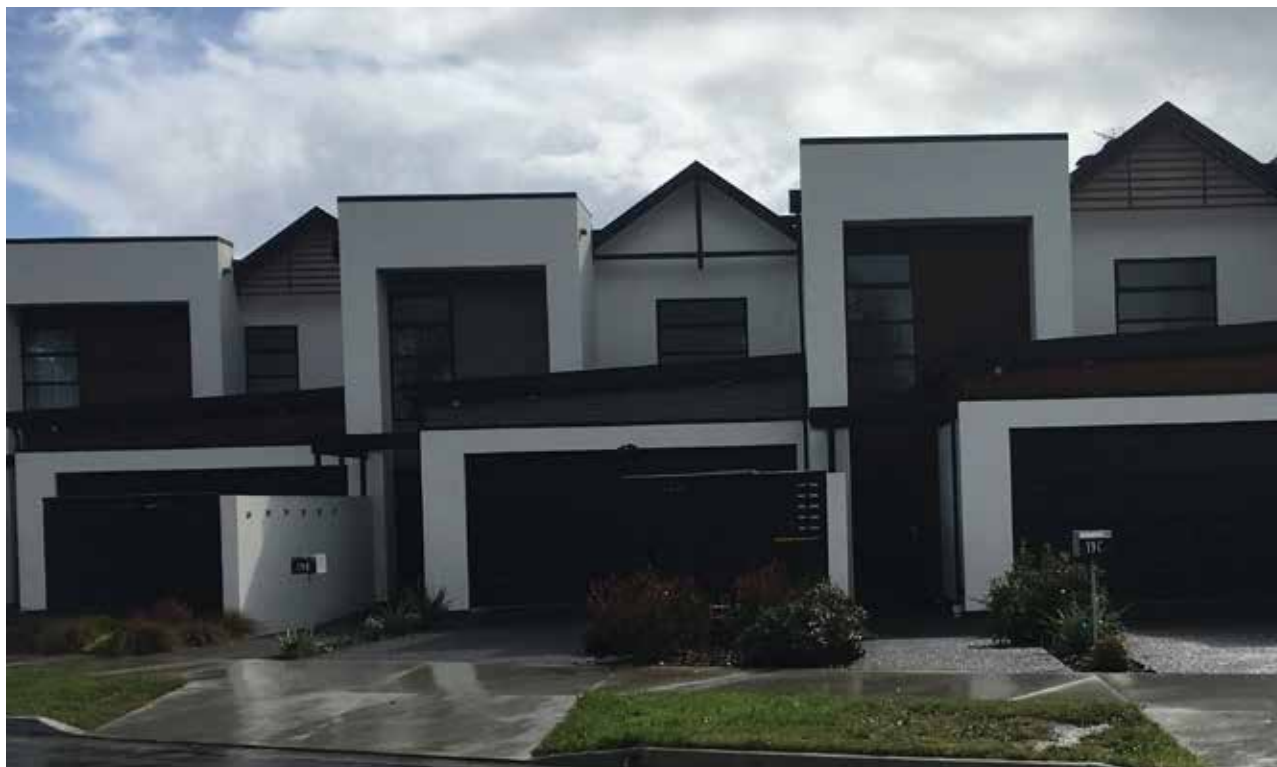
Example : Double garages on narrow sites can lead to visual dominance of garages and poor outcomes for the streetscape, Silverstream Kaiapoi.
