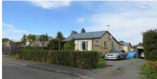
House on Broom Street
