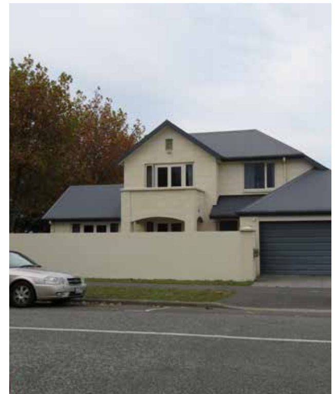
Example : Two storey pitched roof houses in Rangiora.
