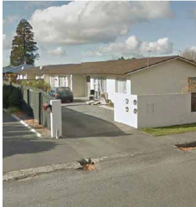
Block of Flats Rangiora.
