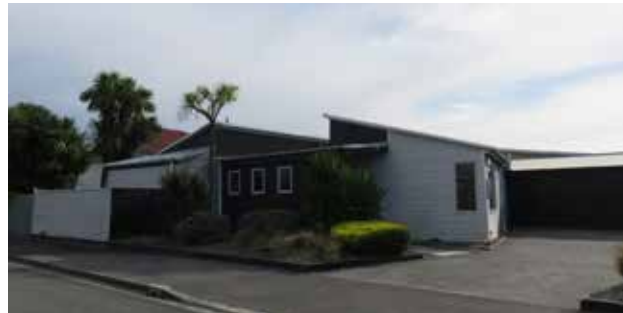
House on Broom Street
