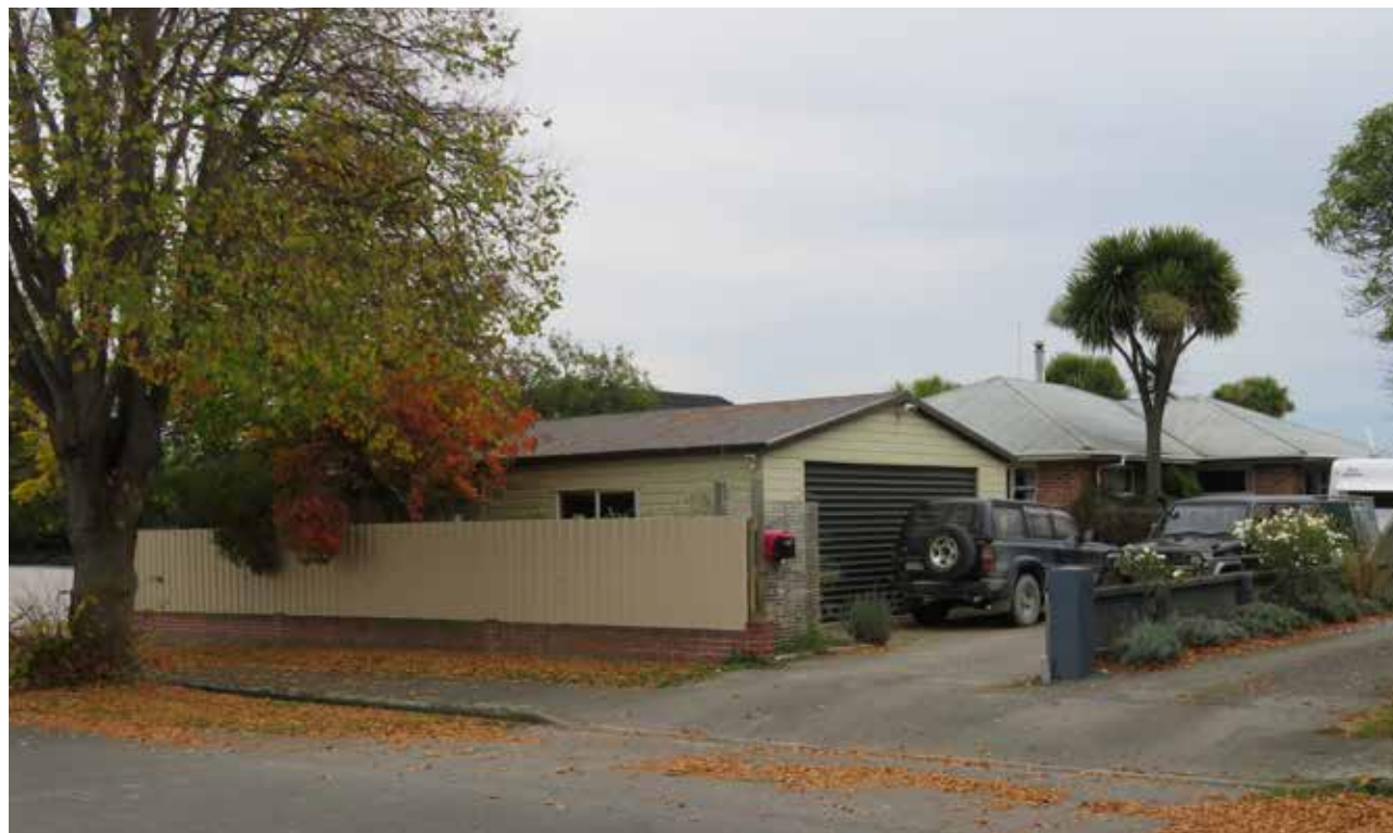
Example : Garage in front garden restricting views between the street and the house, Rangiora.
