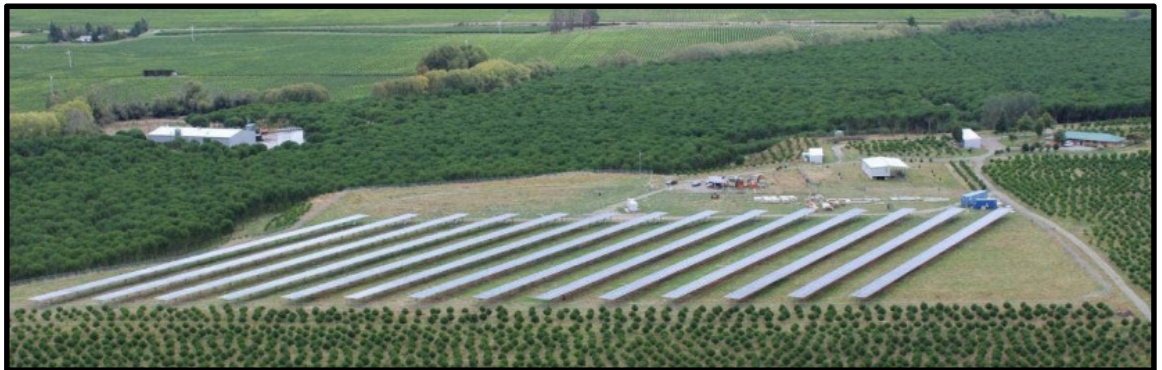
Fig 4 – Example of a single axis tracking solar farm in Marlborough (Annexure D)
