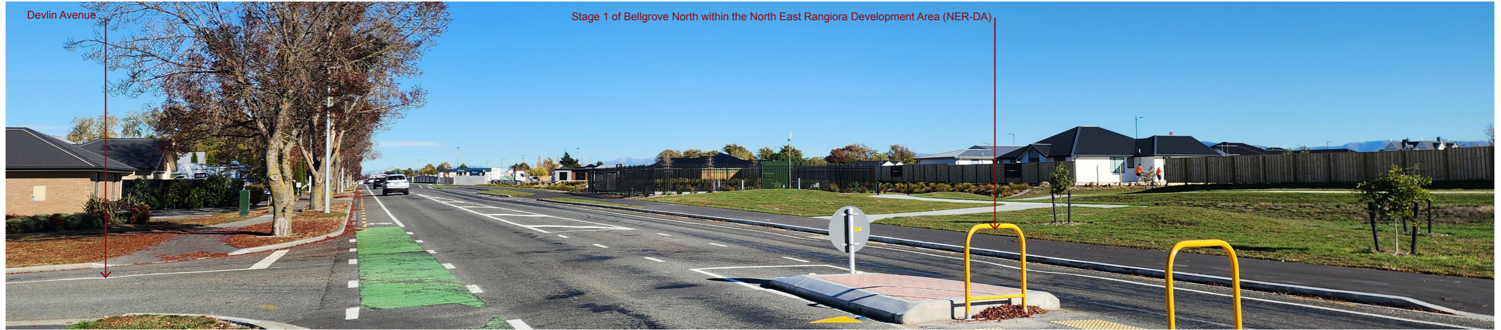
Site Photograph 5: Looking west along Kippenberger Avenue
