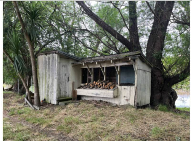
12. Chicken coop along southern boundary line of 144 Main North Road
