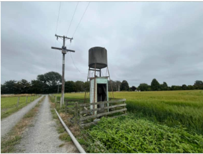
5. Water tank and pump shed at 170 Main North Road
