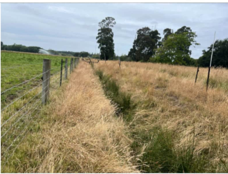
9. Drain/ditch along northern boundary line at 144 Main North Road
