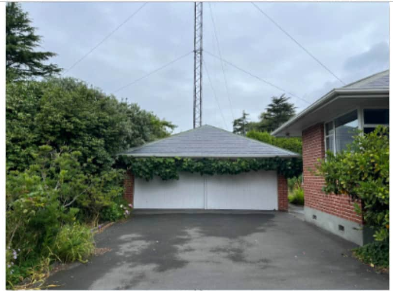
14. Garage at 144 Main North Road
