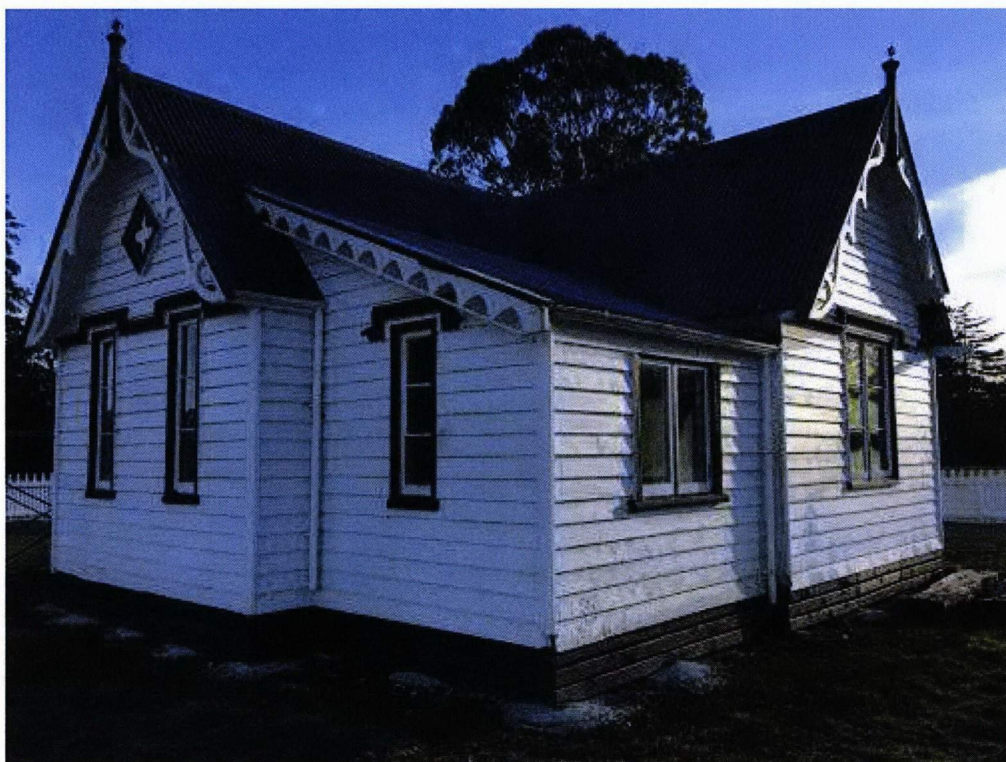
East and south elevations (R. Burgess, 9 July 2019, Heritage New Zealand)
