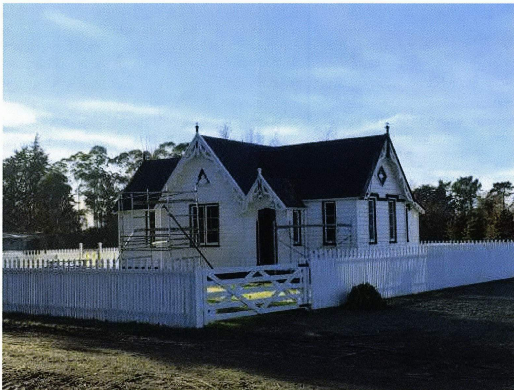
Main (west) elevation fronting White's Road and south gable end (R. Burgess, 9 July 2019, Heritage New Zealand)
