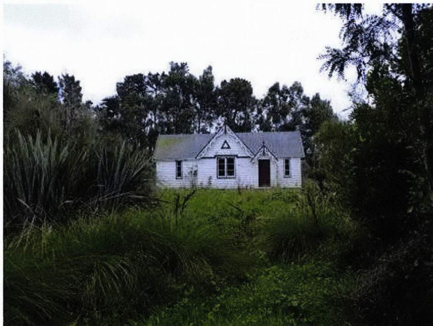
Ohoka Gate Keeper's Lodge (Former) at 127 Jacksons Road , a year before its recent relocation to the Ōhoka Domain (D. Margetts, 12 April 2017, Heritage New Zealand).
