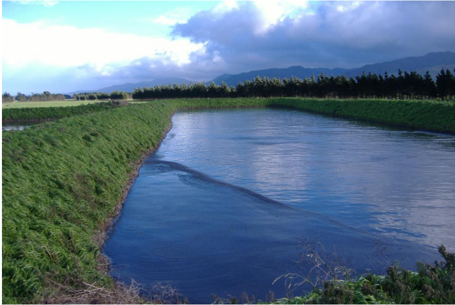
Photo 10: Aerobic pond with reserve storage capacity for winter or high rainfall events
