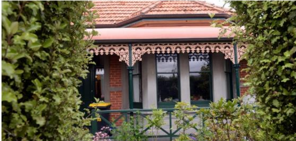
Former Huxtable Residence
