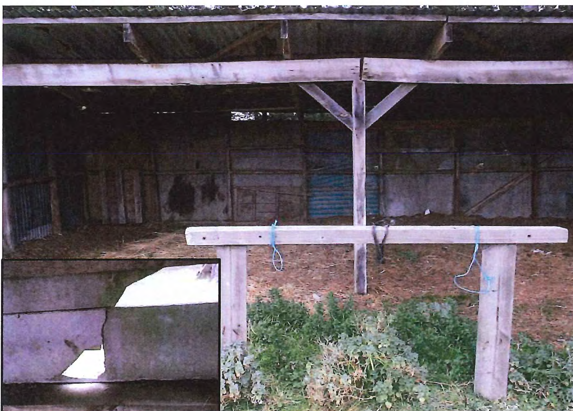
Photograph 12: Property 474 Mandeville Road showing broken cement board sheeting.
